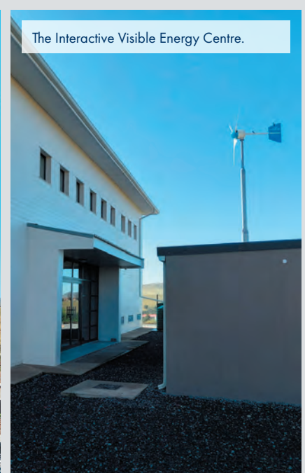
Water harvesting, with the main entrance in the background.
