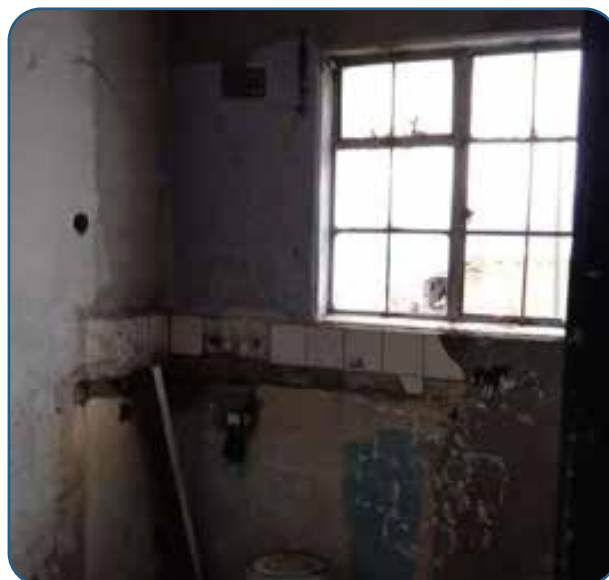
Before the refurbishment work was started.
