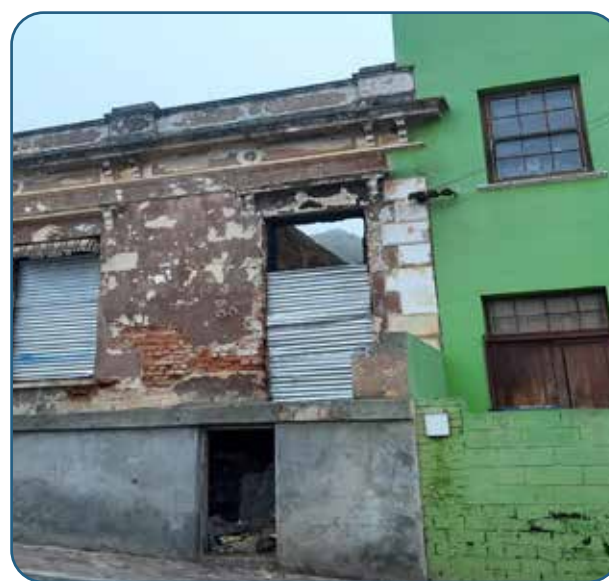
The refurbishment work in progress.
