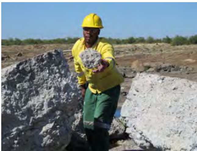
Working for Ecosystems – Removal of dam wall, KNP
