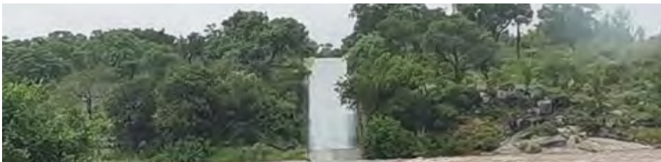
Sirheni Bridge washed away
