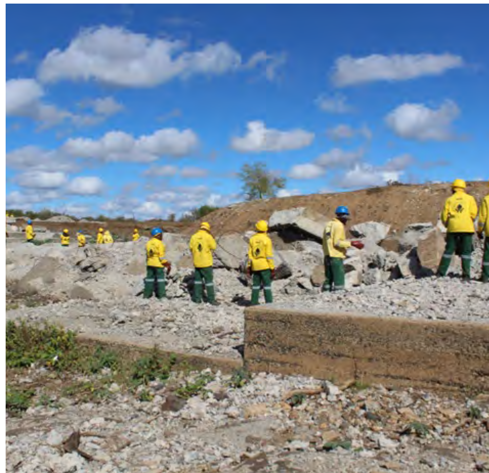
Demolition of Mingerhout Dam
