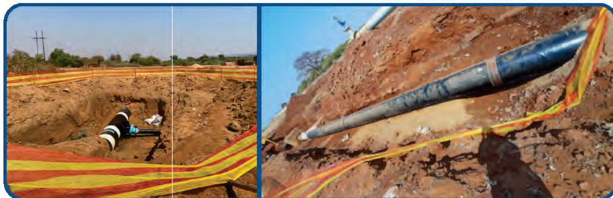
Replacement of the Specon Phase 2 – 2,4 km bulk pipeline within the Olifantspoort Scheme
