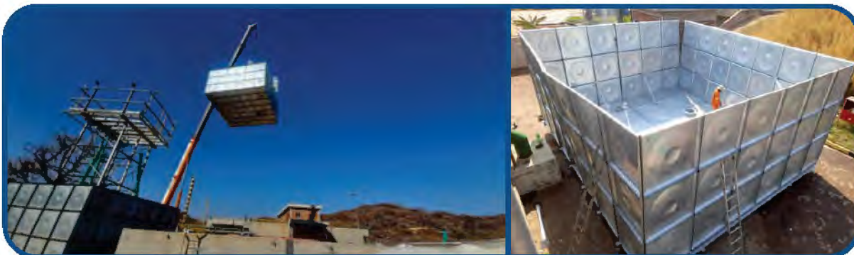
Installation of the Olifantspoort Scheme Service tank
