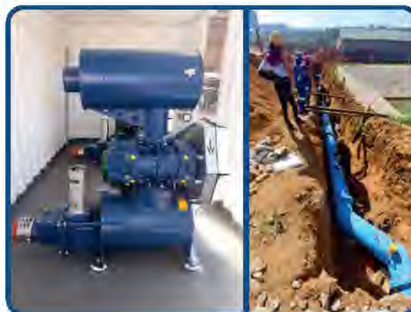
Burgersfort WWTW upgrade and refurbishment project
