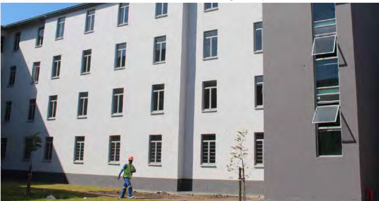
Belhar Project, Cape Town
