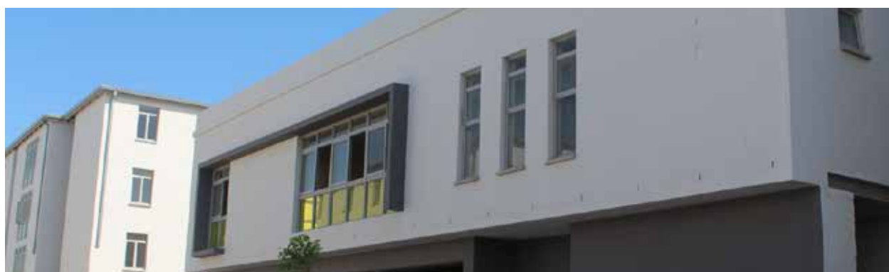
Belhar Project, Cape Town
