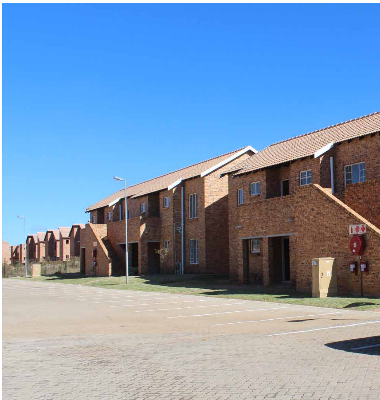
Mogale City Junction, West Rand, Gauteng
