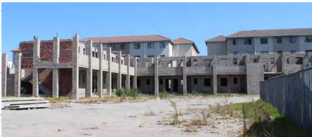
Scottesdene Project, Cape Town
