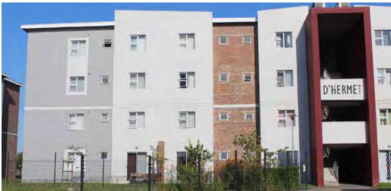
Anchorage Glenhaven Bellville Project, Western Cape
