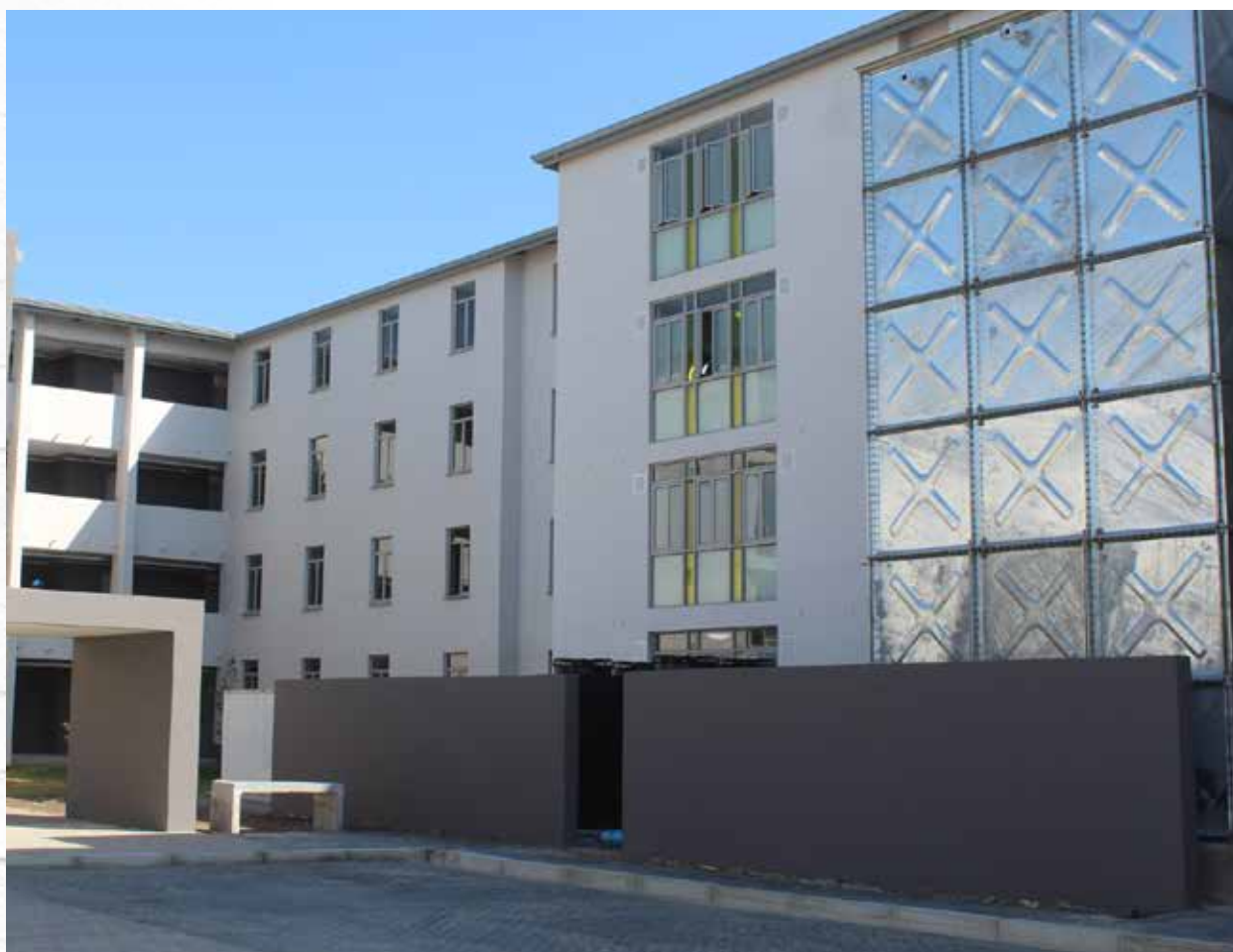
Belhar Project, Cape Town
