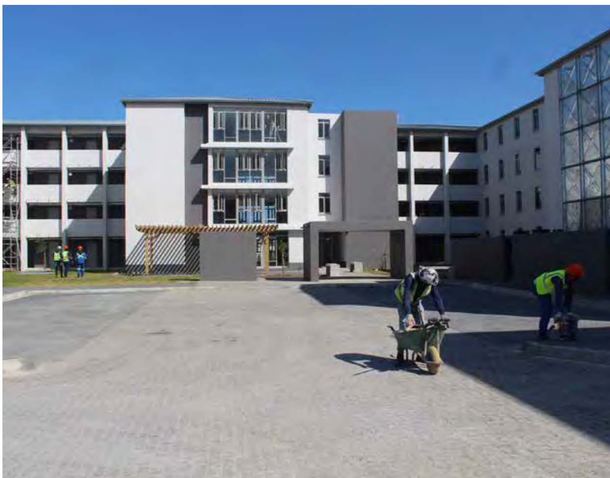
Belhar Project, Cape Town
