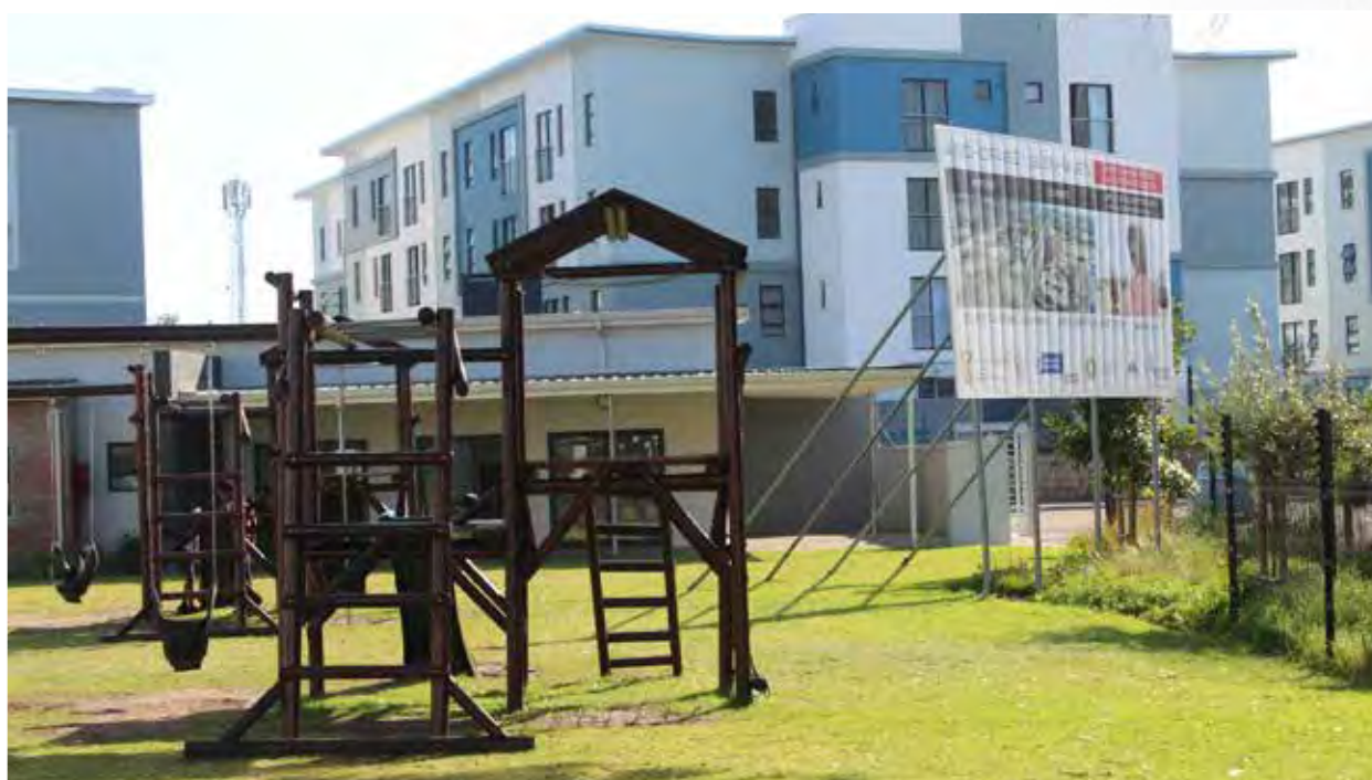
Anchorage Glenhaven Project, Belville, Western Cape
