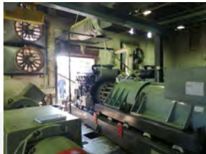
Figure 43: Installation of the Generator
