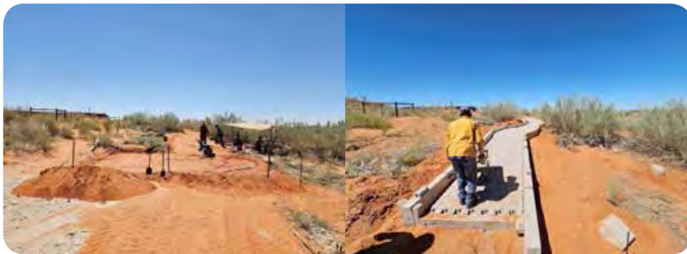
The construction of the new walkway.
