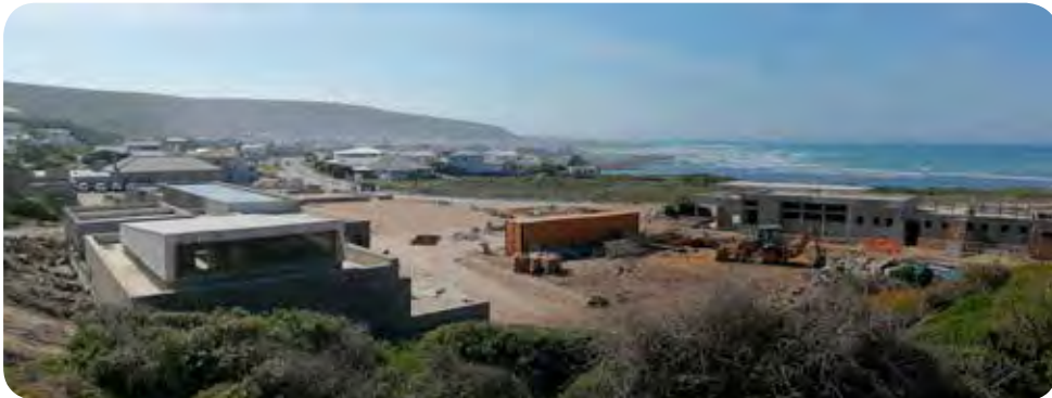
Agulhas Lighthouse Precinct under construction
