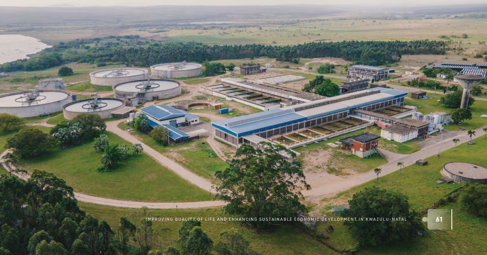
Nsezi Water Treatment Works
