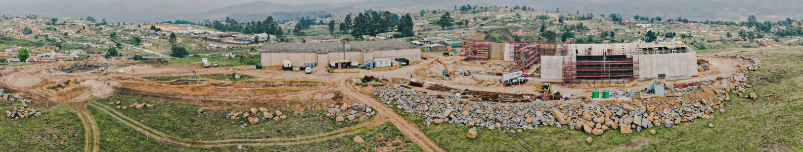
Vulindlela Bulk Water Supply Scheme
