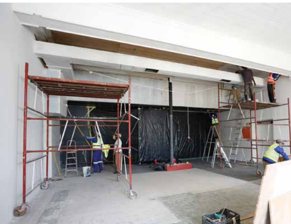
Infrastructural upgrades to the |Qe Power of Rock Art Gallery, Iziko South African Museum, November 2024.
