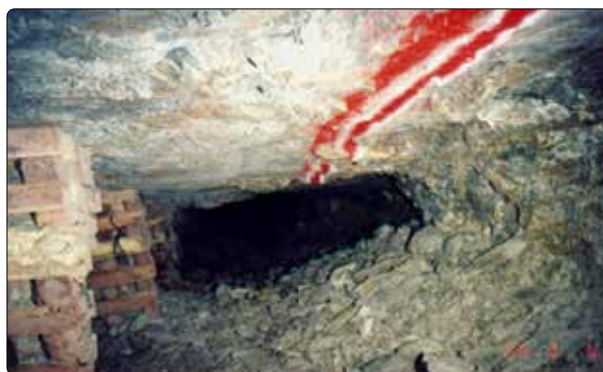
Hangingwall with preconditioning
