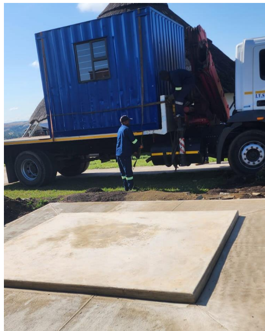
Figure 2. Hazardous Storage Room
