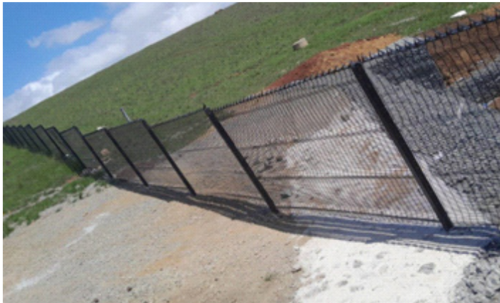
Figure 2. Clear View Fence
