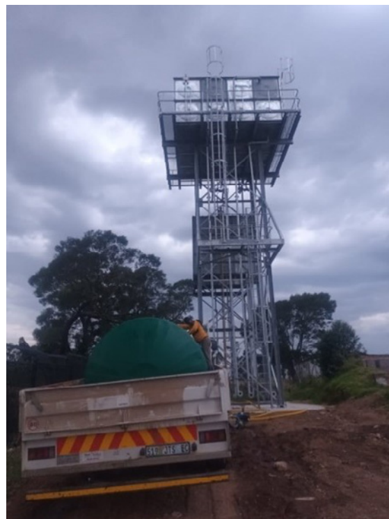
Figure 3. New Elevated Water Tank
