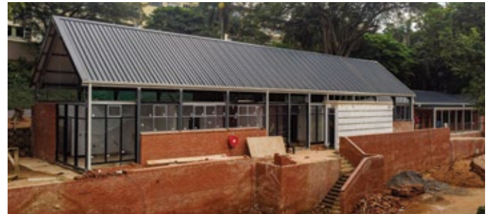
Renovations and refurbishment of buildings at the KwaZulu-Natal Herbarium, Durban.
