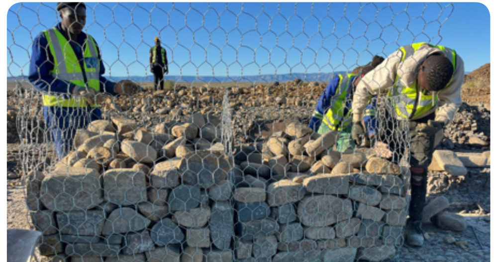
Gabion construction for repair of Oudebaasdamkraal, Tankwa Karoo
