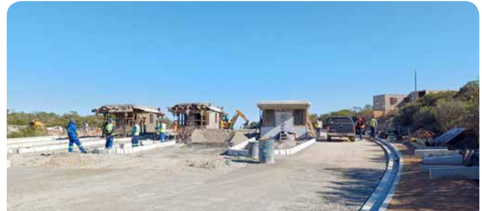
Construction of R27 Entrance Gate, West Coast National Park
