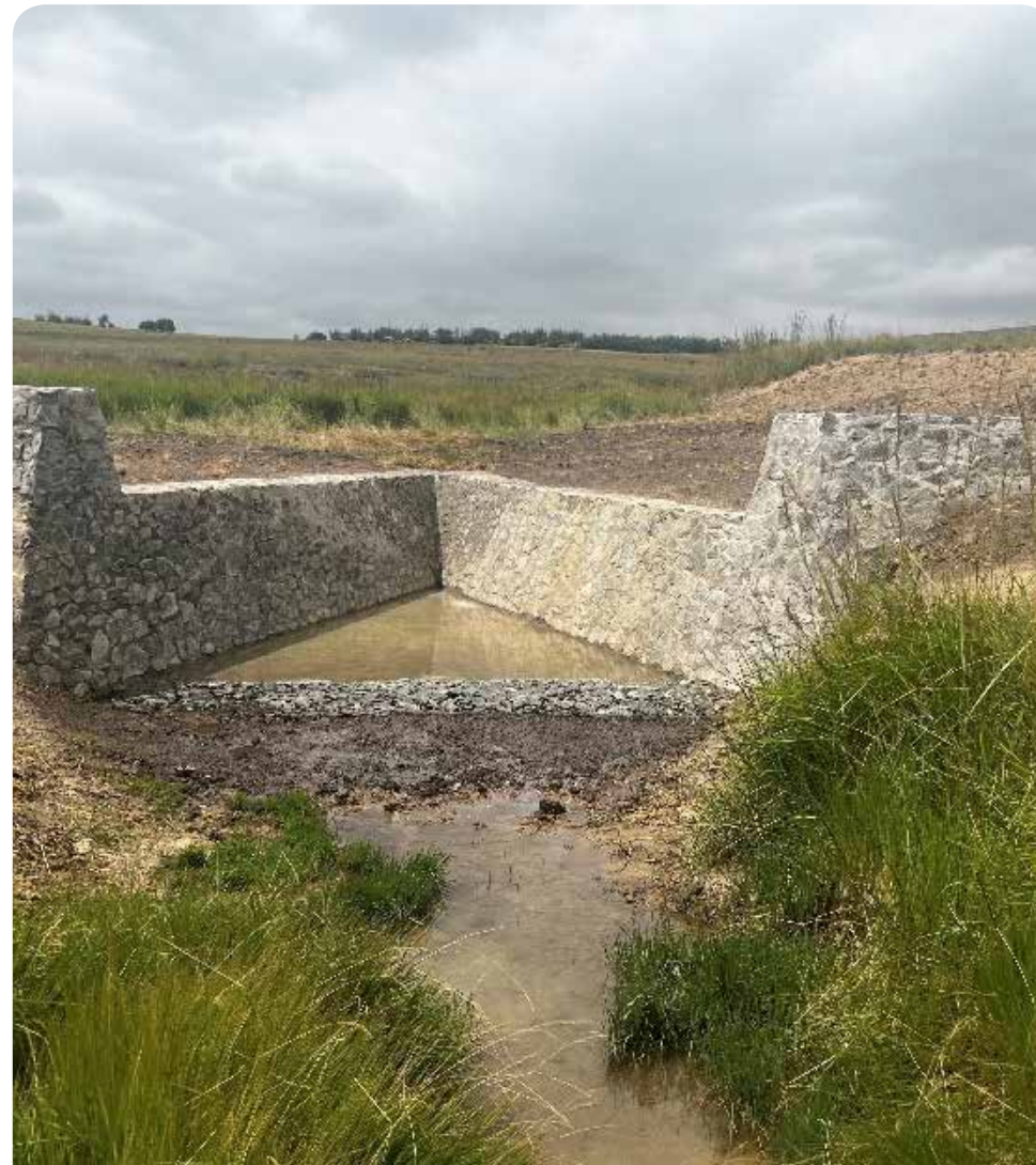
Wetlands rehabilitation in Golden Gate
