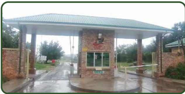
VIMP – Security Entrance upgrade.
