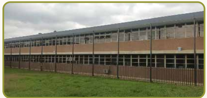
GC Roof Refurbishment and Painting
