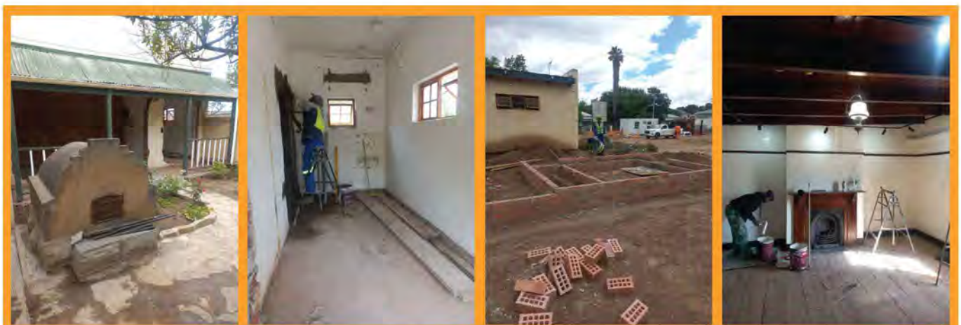
Schreiner House: During the period under review, Amazwi Museums commenced with the Schreiner House Project in Nxuba, the project entailed the restoration and refurbishment of the Schreiner House as well as Ikhamanga Hall. The project is expected to reach completion in the first half of the 2025/26 financial year.
